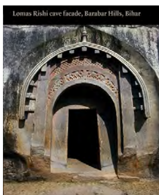
Fig. 2.14b Barābar Hills- The Arched entrance of the Lomas Rishi Cave.
